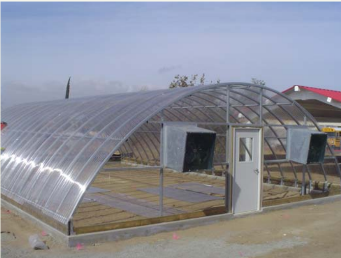
Hemet High Remodel—Greenhouse 2010-11
